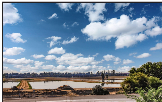
Leaky Acres, a large scale groundwater recharge project in Fresno, is a prime example of what a beneficial land usage could be.
